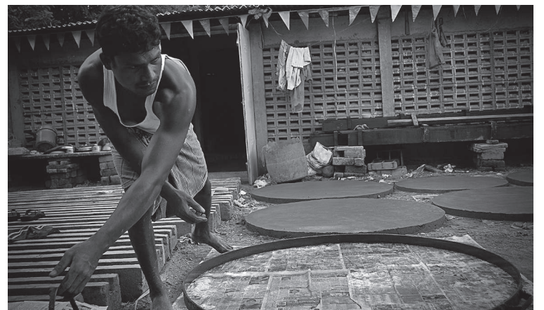
A worker at a cement work factory. Prefab concrete units have become popular as they make construction easier.
